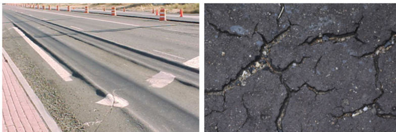
Figure 1: Examples of rutting (left) and cracking (right)
