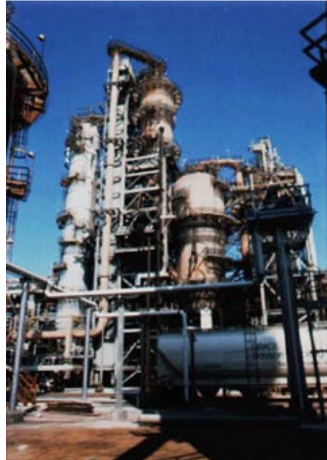
A Fluid Catalytic Cracking Unit. Photo courtesy of Grace Davison.
